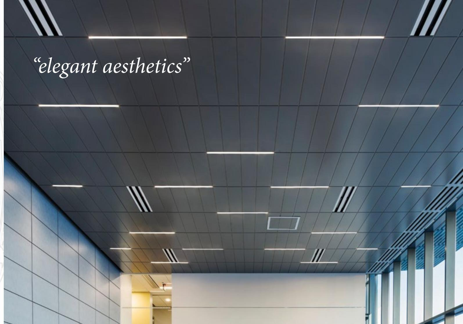
*“The T-BAR LED fixtures were chosen for their elegant aesthetics, ease of installation, and minimal space needs in the ceiling plenum.”*
