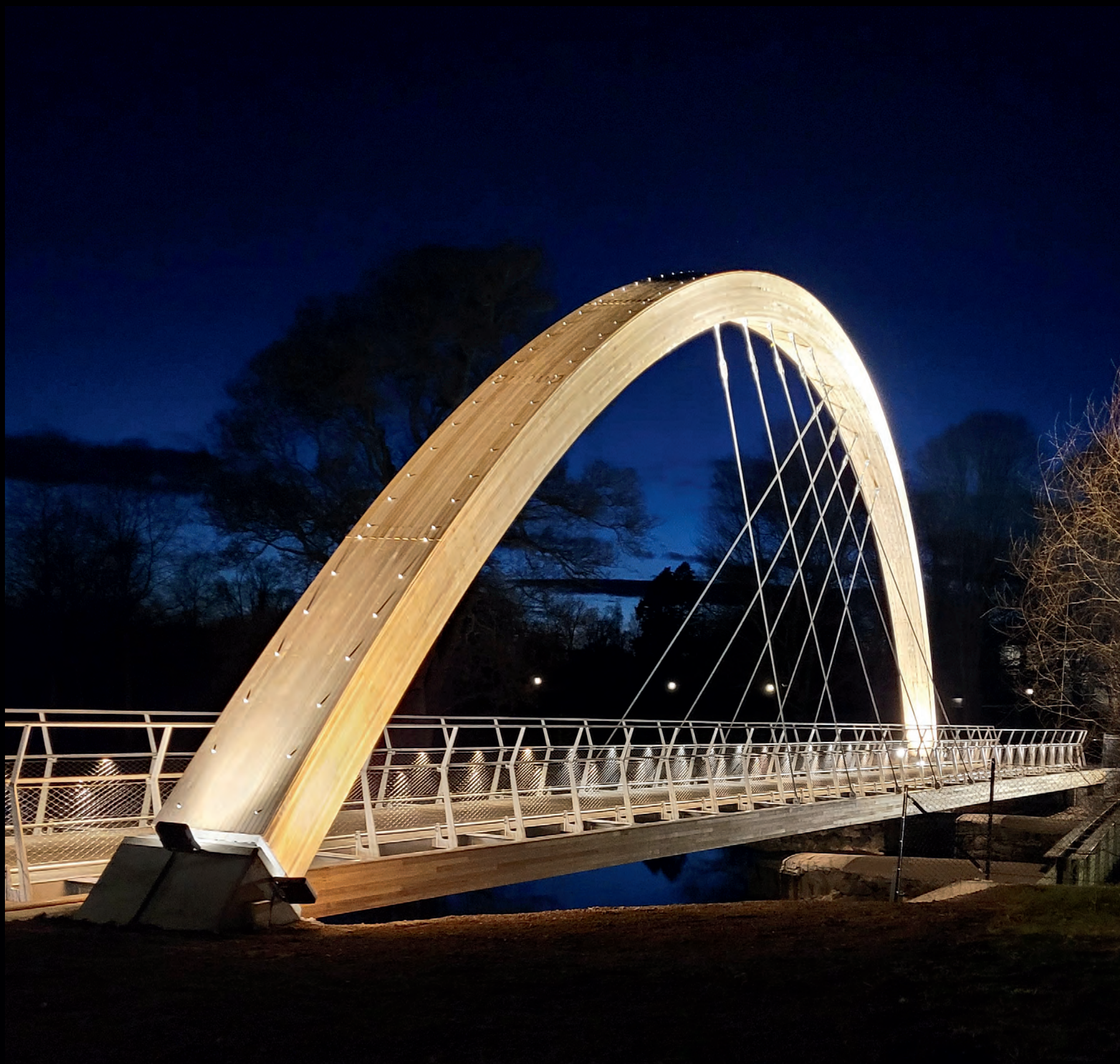
Sweden – Björkbornsbron Bridge, Karlskoga
