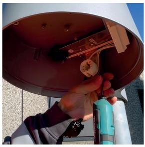
Unfasten the plug and remove the base plate.
