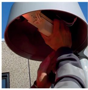
Press the LED module into position and connect the plug.
