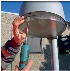
Remove the diffusor by means of 5 mm hex key. If required, the diffusor can be removed from its base in horizontal position.
