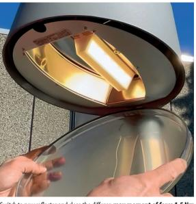
Switch to new reflector and close the diffusor, max moment of force 1.5 Nm
