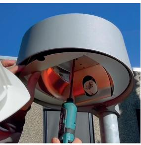
Remove the lamp before removing the reflector.
